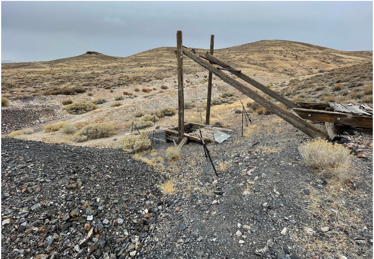
Figure 6. Historic Silver Coin headframe near utm N4531058 E472347. At this location, dump material is silicified, quartz veined, oxidized (limonite > hematite) and variable amounts of carbon. Exposed in the roadcut behind the headframe is weakly oxidized and bleached igneous material of the Iron Point intrusion.
